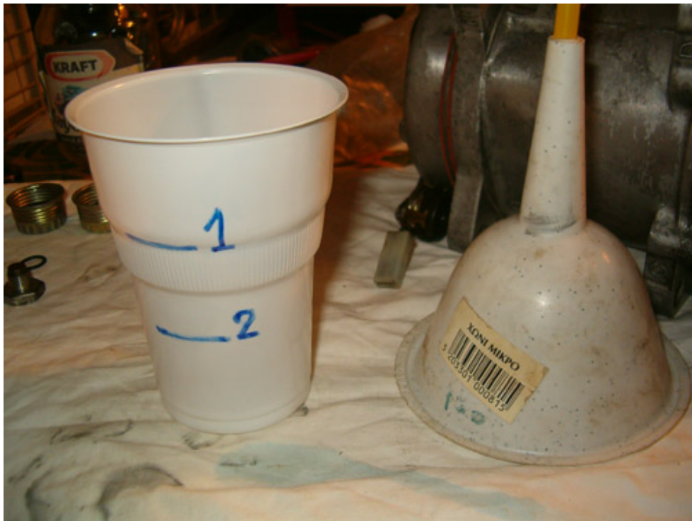
... and using a suitable funnel, pour it slowly to compressor body
